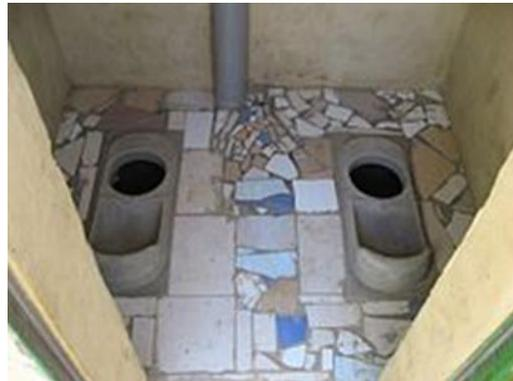
All UDDTs were built entirely above ground to facilitate the air circulation in the vaults/buckets, thus accelerating the drying process. The toilet buildings have a small staircase (2 to 3 steps).
