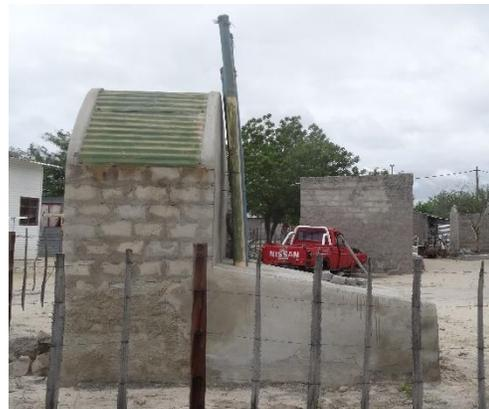
For the provision of improved sanitation, the project introduced dry toilet systems. Different designs of waterless toilets were obtained and demonstration models constructed at community centres. After residents weighed pros, cons and costs of each design, a preferred model was selected. The selected model convinced by being odourless, and from this derives its acronym 'okakedi' toilet, standing for okanjuwo kakena edimba ('non smelling toilet').
