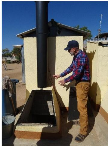
Back view of the Otjitoilet, with ventilation pipe and open chamber where the perforated containers are positioned.
