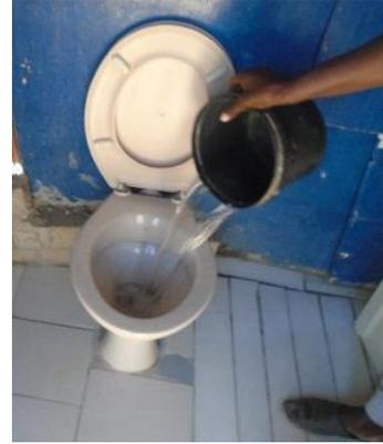
'Normal' toilet seat on pit latrine, floor with tiles, and used in combination with pour flush system (Havana, Windhoek)
