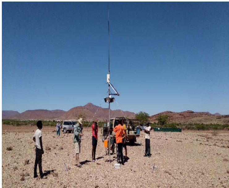
RRT erecting EW tower at Okaturua, Anabeb
