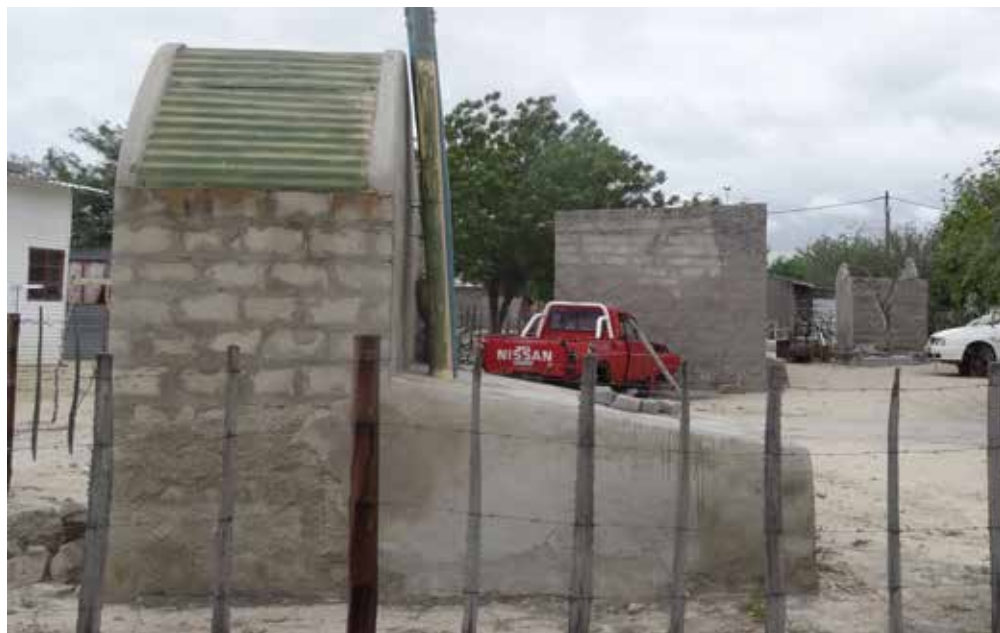
A typical pit latrine design found in many of Oshakati's informal settlements.
