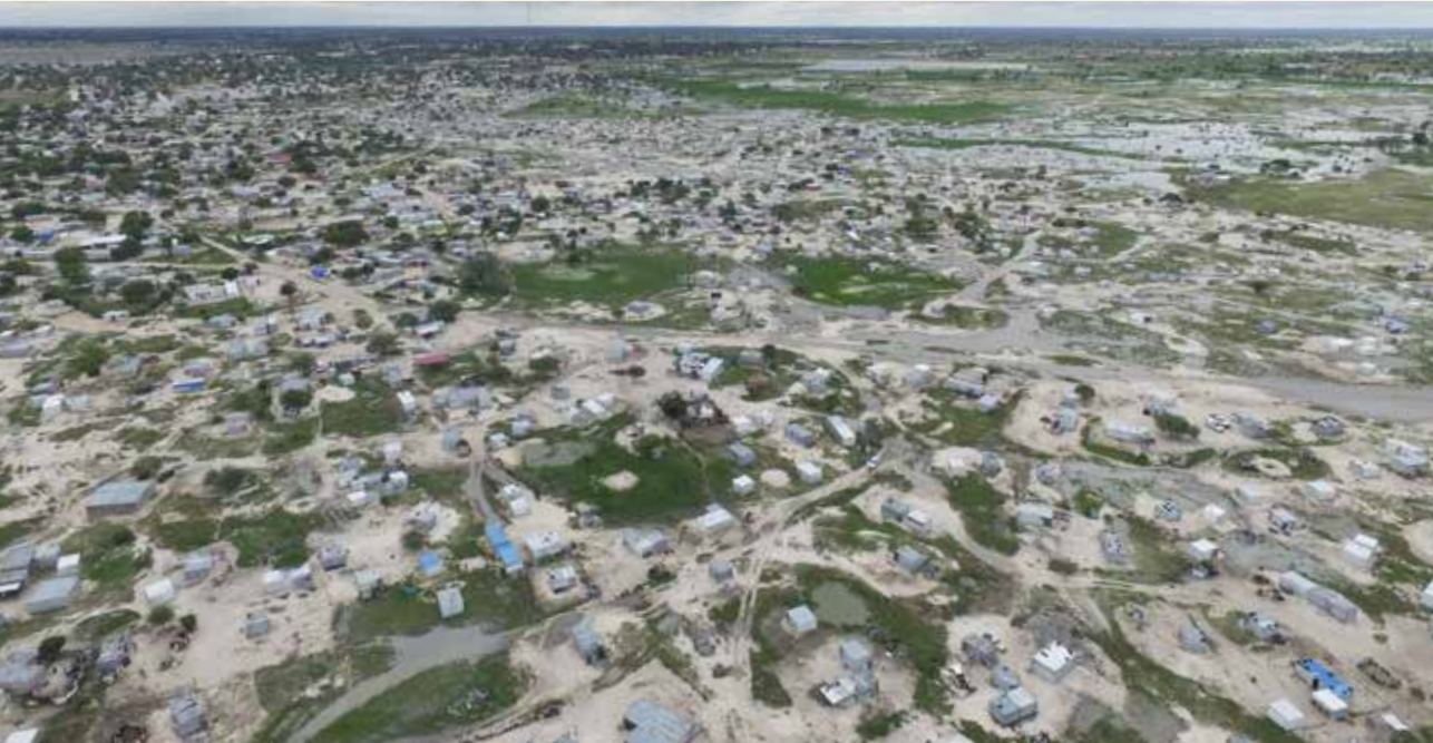
Aerial view of Uupindi South where new shacks have been constructed over the last years.
