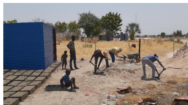
Brick construction of a new plot owner in Oshakati
