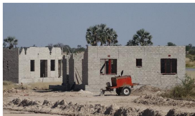
New homes being built in Okahao
