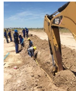
Water pipe installation, Okahao, phase one
