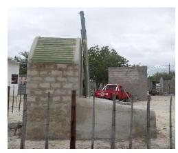
For the provision of improved sanitation, the project introduced dry toilet systems. Different designs of waterless toilets were obtained and demonstration models constructed at community centres. After residents weighed pros, cons and costs of each design, a preferred model was selected. The selected model convinced by being odourless, and from this derives its acronym 'okakedi' toilet, standing for okanjuwo kakena edimba ('non smelling toilet').
