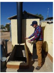
Back view of the Otjitoilet, with ventilation pipe and open chamber where the peforated containers are positioned.
