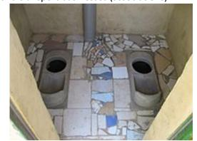
time for the feces is about 6 to 8 months. However, two vaults of this size can normally cater even up to 15 persons. Construction cost are equivalent to N\$ 4,324, of which 61% subsidized by project and 39% paid by end user.
